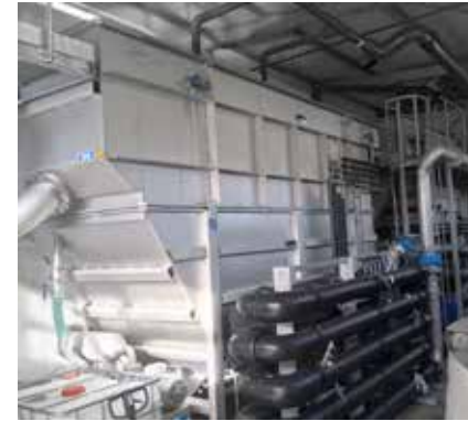
HUBER Dissolved Air Flotation Plant HDF for grease and solids reduction prior to indirect discharge.
