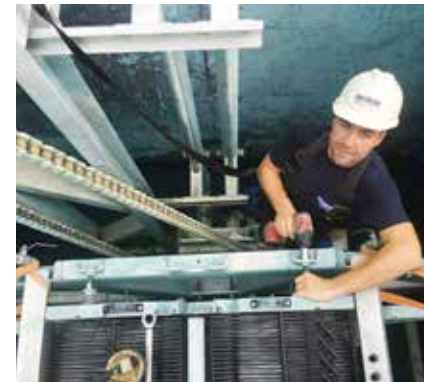
Successful start of operation due to professional installation.
