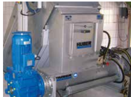
HUBER Wash Press WAP® installed behind a HUBER Fine Screen STEP SCREEN®.
