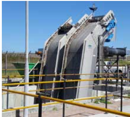
Robust screen for coarse material removal: HUBER Coarse Screen TrashMax®.
