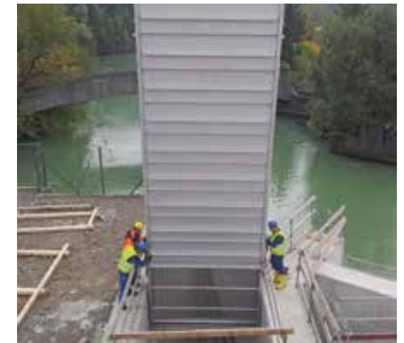
River water screening with the HUBER Multi-Rake Bar Screen RakeMax® V for high volumes of wastewater.
