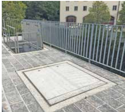
Load bearing HUBER Manhole Cover SD7.
