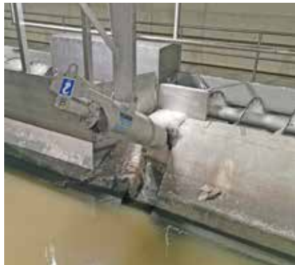
HUBER Storm Screen ROTAMAT® RoK1 TS for the reliable removal of screenings.
