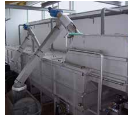
Complete mechanical wastewater treatment in a single and compact unit.
