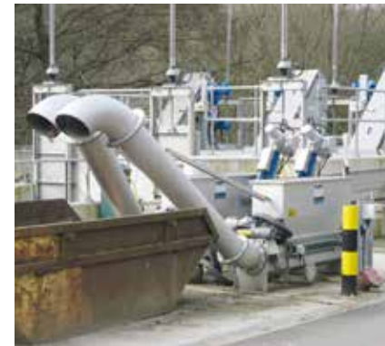
HUBER Wash Press WAP® L with launder channel feeding system: redundant operation and optimal screenings dewatering.
