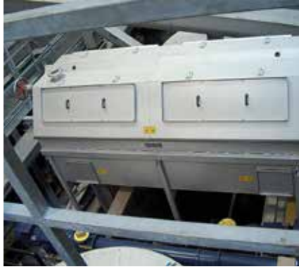
HUBER Drum Screen RoMesh® for fine and finest material removal.
