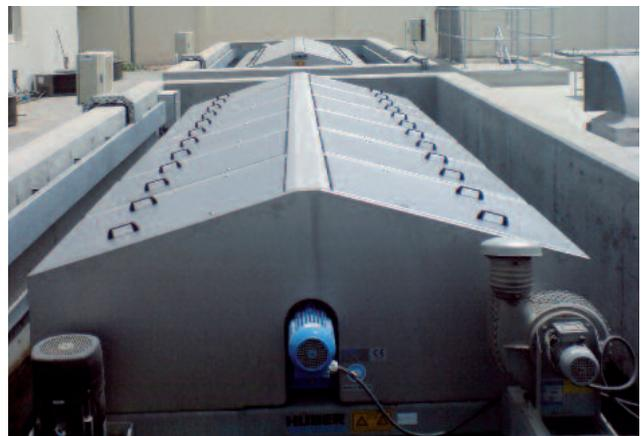
*RoDisc® Rotary Mesh Screen with 20 discs installed in a concrete tank*
